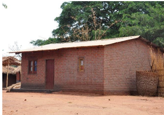
Figure 8 – Iron sheet roof. Abadia (2016)
