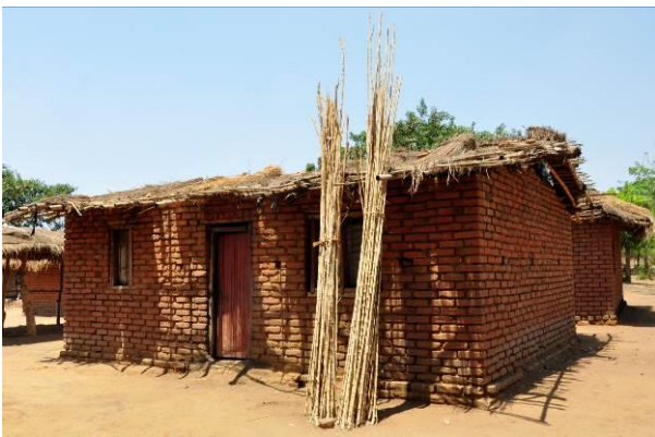
Figure 7 – House with a grass roof. Abadia (2016)
