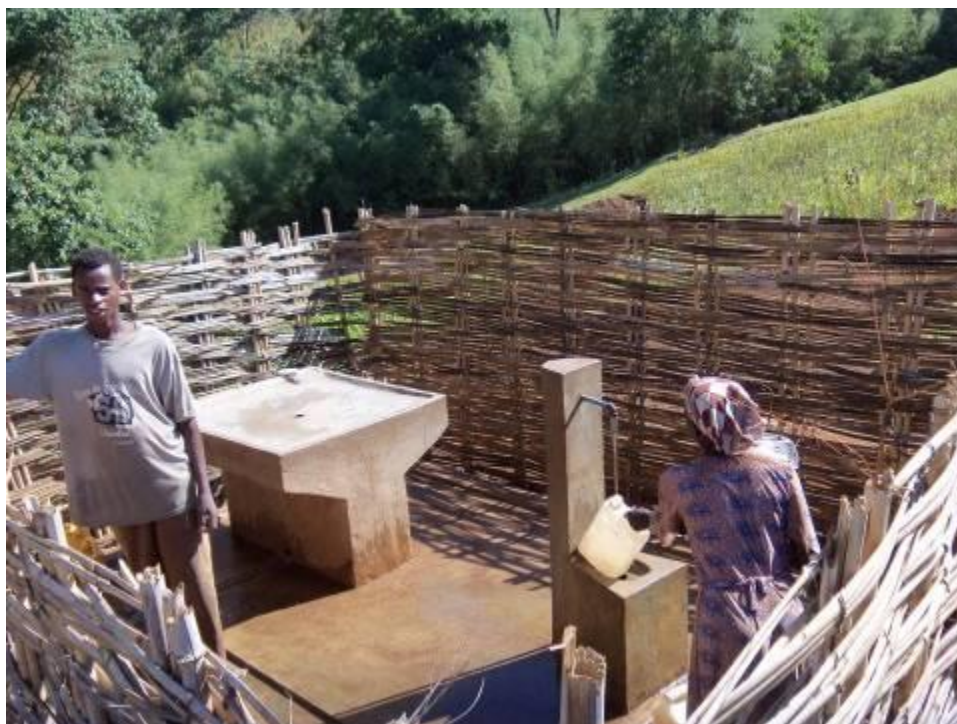
Pic-7 A typical arrangement for a water point & cloths washing basin at a water facility. Mareka
