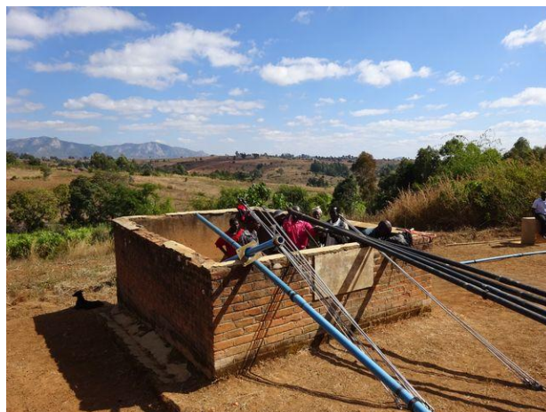
Repair of a borehole
