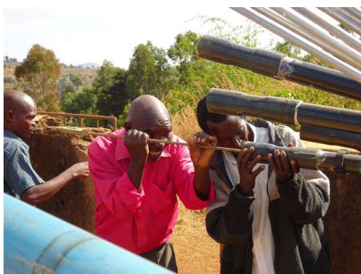
Two area mechanics joined for this difficult repair
