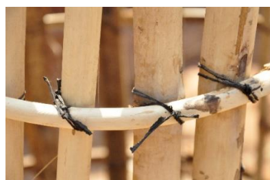
Posts are tied with inner tubes. Abadia (2016)
