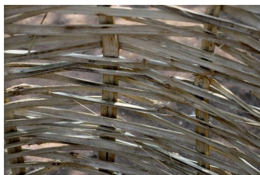
Bamboo strips weaved around bamboo posts. Abadia (2016)
