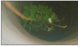
**4.** Make the **candle test** (as you see in the picture you tie a candle to a rope and you put it down lighted into the well: if the light goes off, it means there is not enough oxygen, you need to wait)
