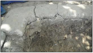
If the surface work was done with **no** reinforcement (soak away pit on the top) or with a **poor mixture** (apron on the right), after few months, several cracks will progressively appear.
