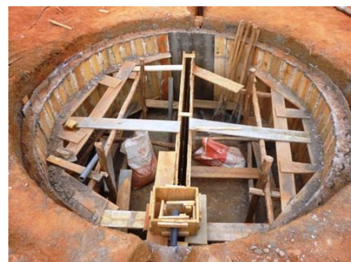
Reservoir with 2 compartments under construction
