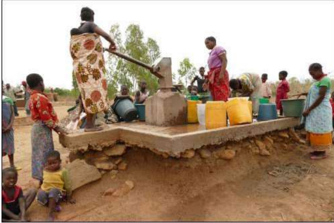
Figure 1: a water point with an apron built about 10 years ago. The eroded soil under the apron is estimated about 50 cm; the erosion rate per year is there- fore estimated as 5cm/y.
