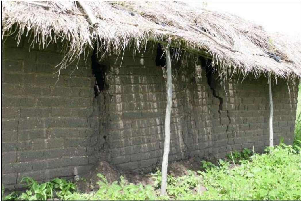
Figure 4: a house build with mud bricks and temporary roofing is going to collapse, due to the melting of the bricks, after 2 days of rain. As deforestation progress, this kind of bricks are more and more used for “non-shelter” building such as toilets; the poorest class of the rural population use them even for houses.
