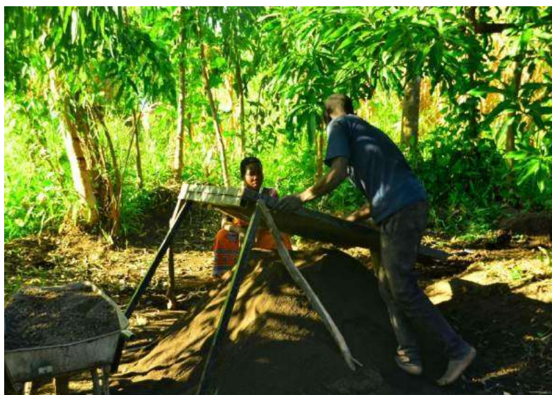
Figure 10: a beneficiary family is sieving the necessary soil for the bricks.
