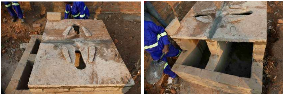
Figure 19: the chamber building with its two slabs
