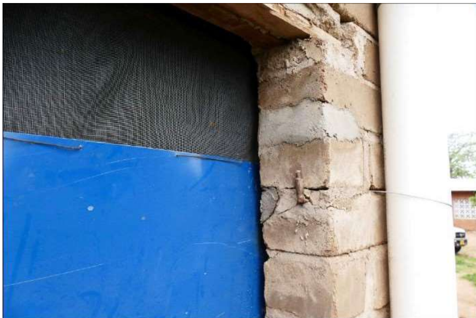
Figure 30: the door has been installed with internal hinges, not visible to the public, in order to make possible theft/vandalism more difficult. (The visible hinge at the wall is not any-more relevant).
