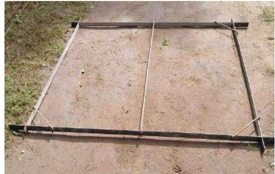
Figure 5: footing mould used to build the base of the toilet.
