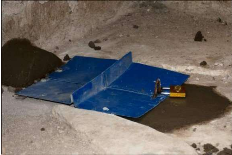
Figure 31: the two holes of the slabs are provided by a lock, in order to allow the students to use only the correct side of the chamber, letting the teachers to choose when it will be the right moment to shift the chamber side.
