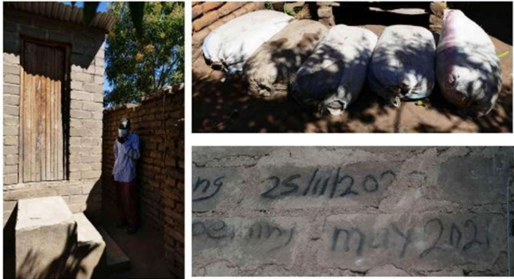
Figure 36: the beneficiary is showing the toilette of his house, the new 5 bags of manure collected from the first chamber, and the date of closing the first chamber written inside the toilette.
