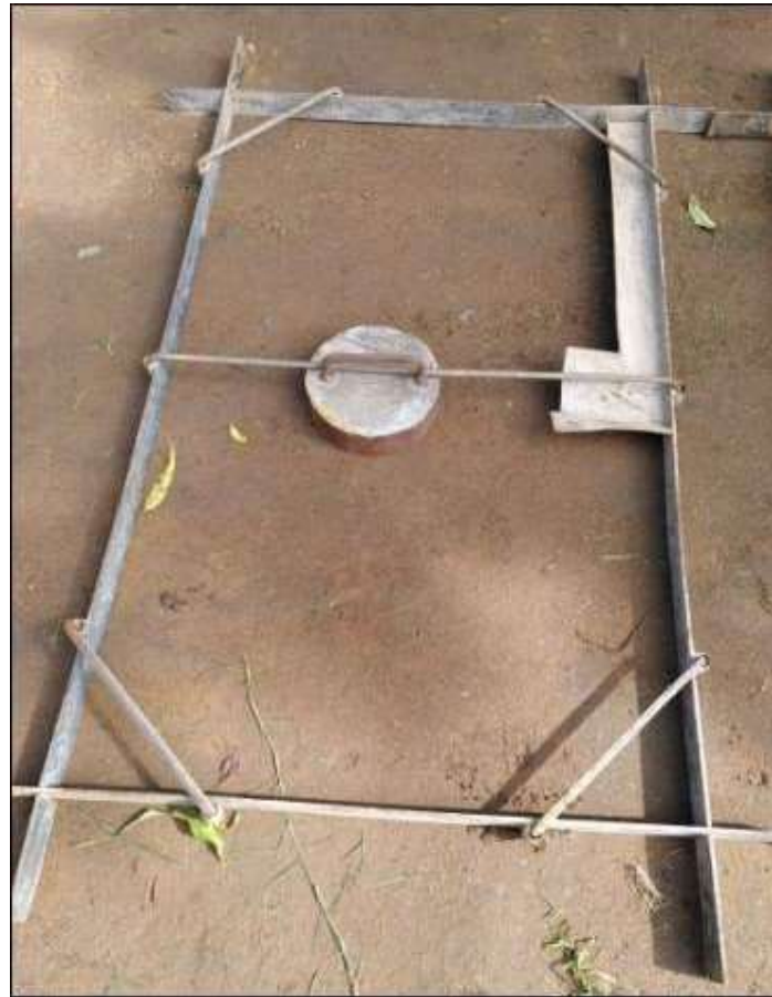
Figure 9: slab mould, with its welded urinal channel and hole-rounded mould
