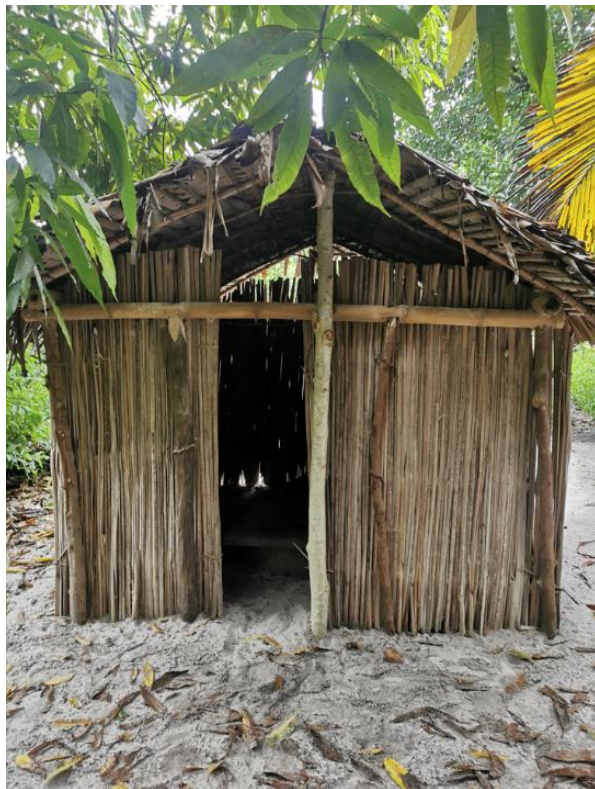
Double pit latrine at Tanambao, Analanjirofo
