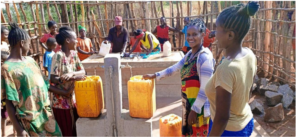
A water point in use: drainage below the taps going to the cattle trough, wash table at waist height.
