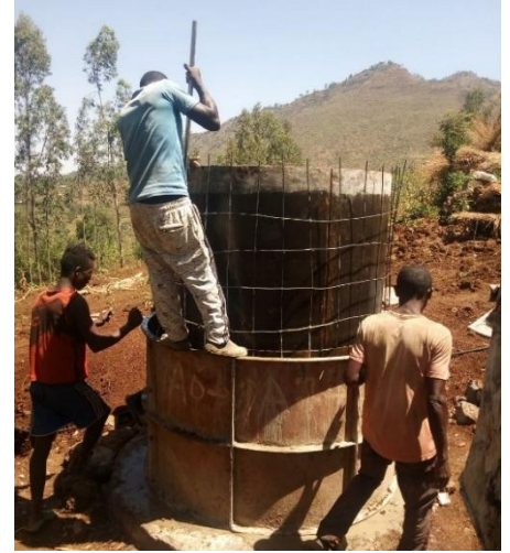
A reservoir under construction in its metal mold.
