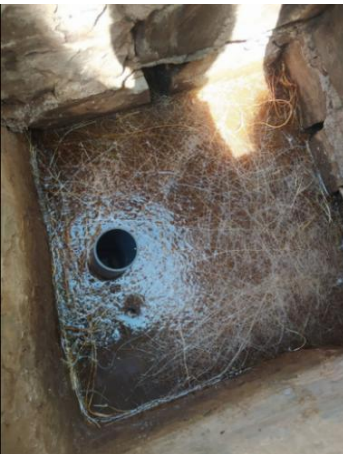
What an uninspected spring box looks like inside: root growth left to develop unchecked
