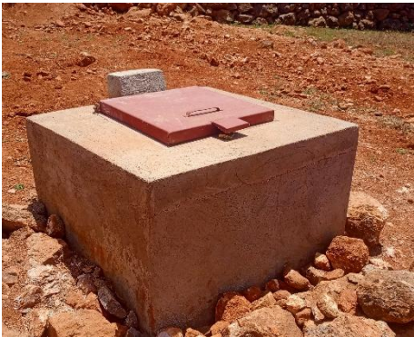
The distribution box splitting flow in proportion to outlets diameter.
